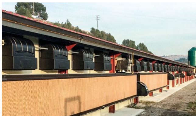
TPI Polytechnik's wind hoods made in polyurethane are used, e.g., in poultry houses.
