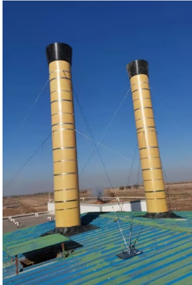
TPI Polytechnik's chimneys installed on a pig farm in China
