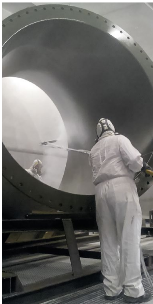
Applying Accosshield corrosion protection coating
